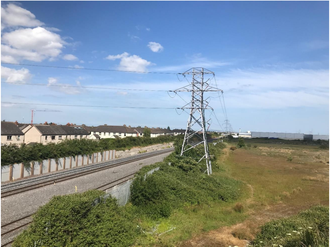
Photo 3: View of Northern Boundary of the Site with Dublin to Cork Mainline Railway
